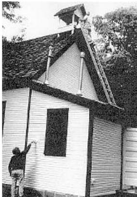
time and limited finances have permitted. Much of the necessary demolition work has been completed, structural repairs on the roof trusses and ceiling rafters have been accomplished, and some new drywall has been installed. Much remains to be done, however.
