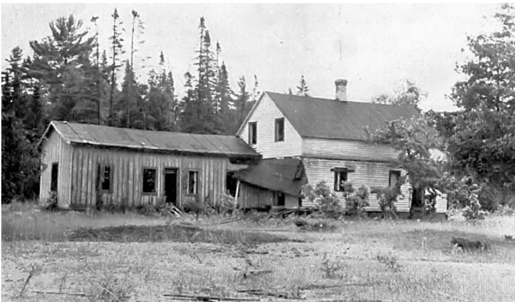
Back in the days when this island was a bustling lumbering community there was an up-to-date boarding house. Here it is today, but choked by the encroaching forest. Natives are rapidly demolishing it however, using its lumber for repairs to homes.
