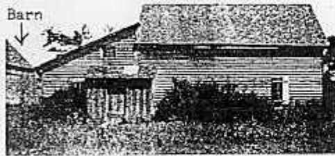
The old Hutzler home shortly before it was torn down.
