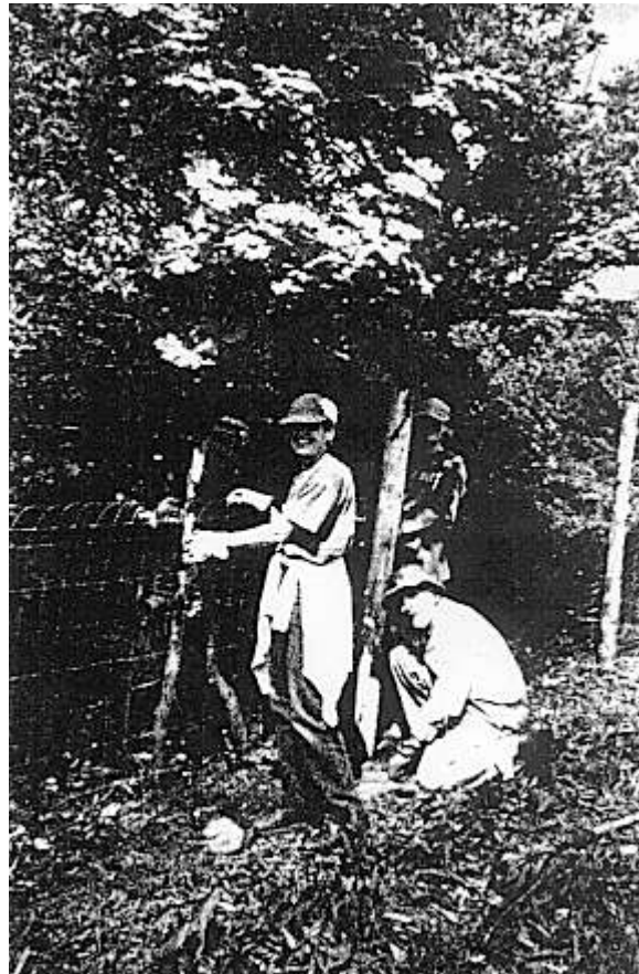
"Smiling and Building the Fence" South Manitou Island Cemetery
